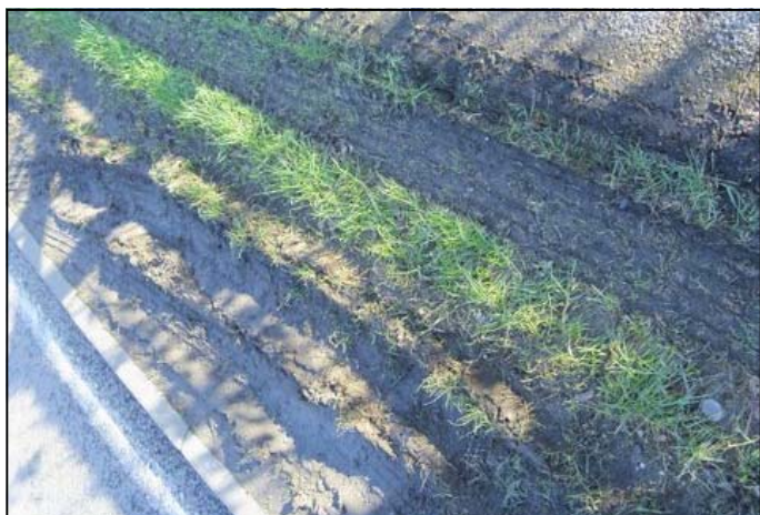
Above: Tyre damage caused to the grass verge on Lower Luton Road by heavy vehicles
