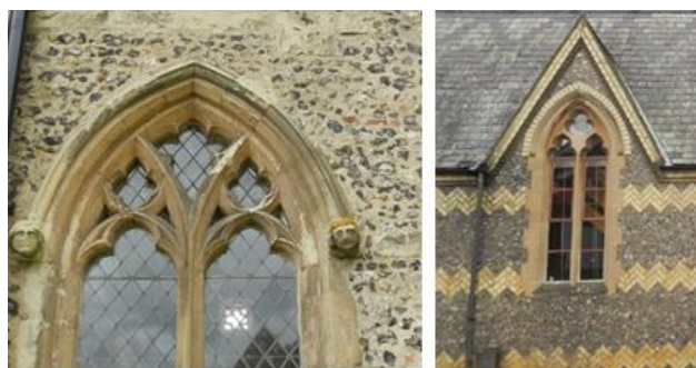
Windows at St Helen's Church and Old School House
